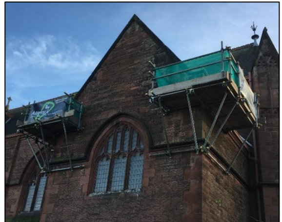
Suspended scaffolding above the north-west stairwell gable.
